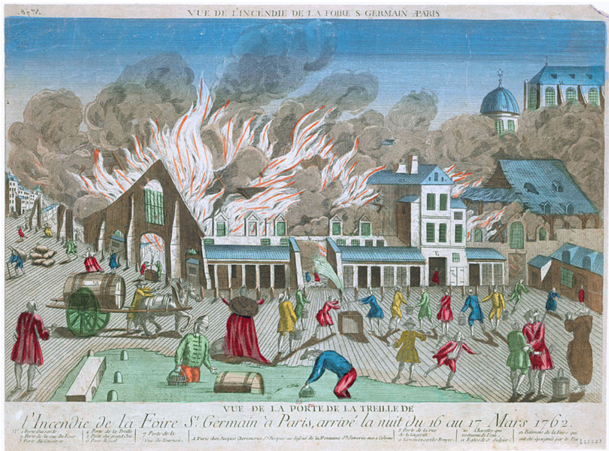
Figure 1 Jacques Chéreau, “Fire at the Saint-Germain fair” (1762). © Gallica.bnf.fr. The bucket chain and fire pumps are clearly visible. A water cart is approaching on the left and a monk is present on the right.
